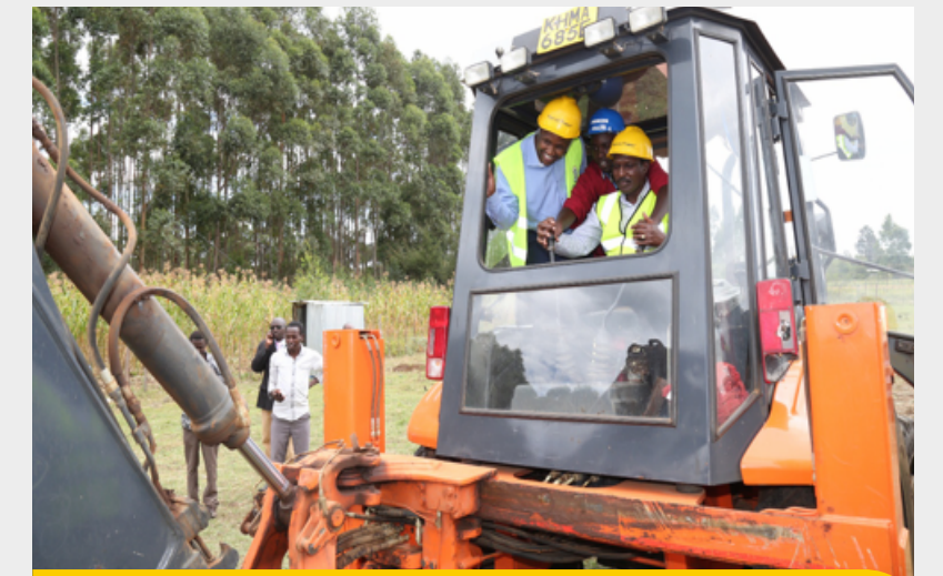
Ground-breaking of Olessos Stima School, Nandi County
