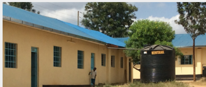
Renovated classrooms at Muvwana Primary School in Mwala, Machakos County
